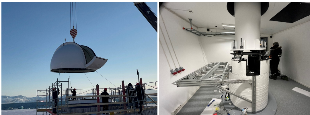
Figure 7. The dome (left) and riser and optical bench support structure (right) was installed in the Ny-Ålesund SLR shelter in March 2022. Photos: Gøril M. Breivik
