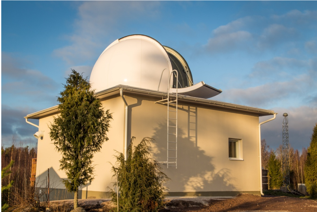
Figure 1. The new SLR building of the Metsähovi Geodetic Research Station.
