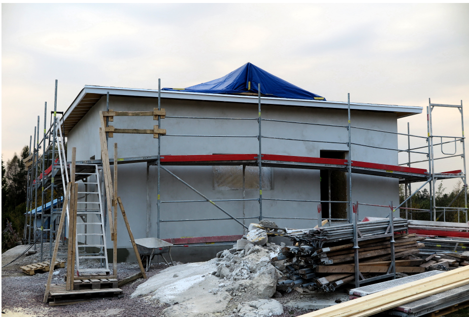
Figure 4. New SLR observatory building being built at Metsähovi, October 2014. Photo: FGI
