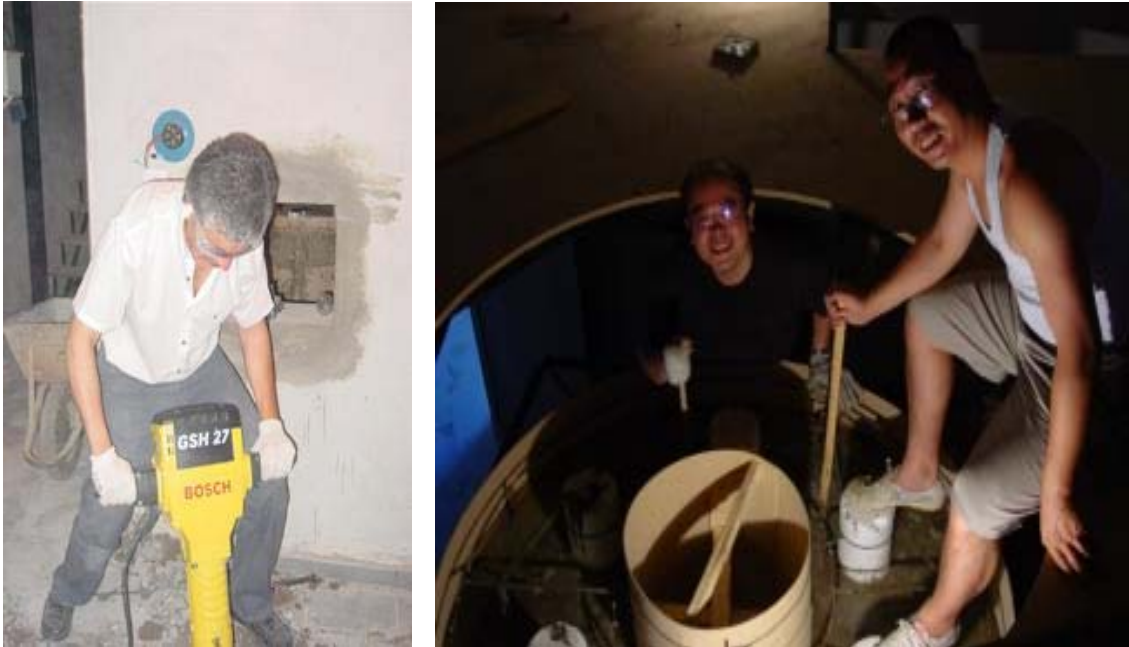
Figure 4: Base of laser platform and Base pillar of the telescope modifying
