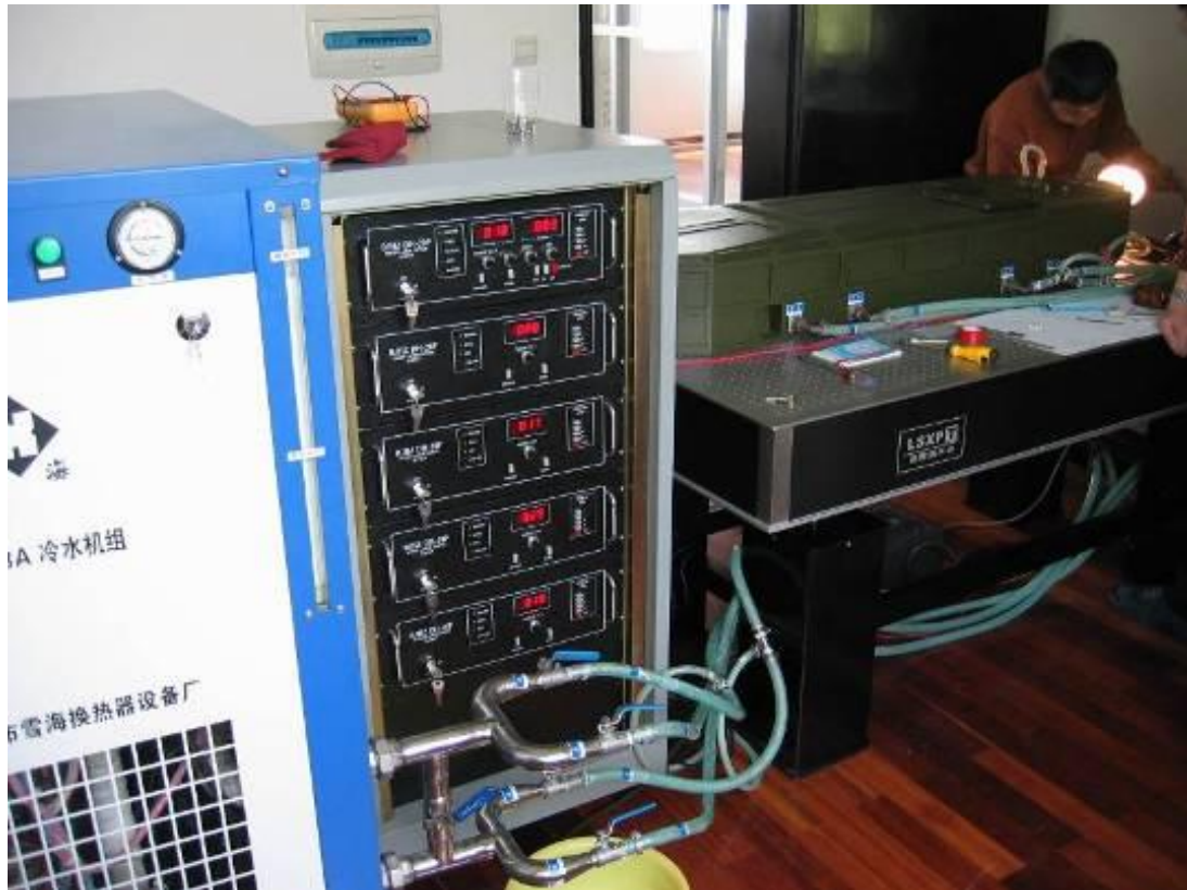
Fig.5. High Power Laser & Power Supply, Chiller
