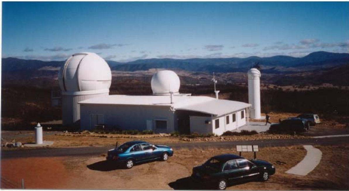
Figure 1: View of the EOS Space Research Centre on Mount Stromlo, taken from the North-East calibration pillar. The 1.0-metre SLR telescope is inside the Typhoon-III dome atop the main building. The large Icestorm dome houses a prototype 1.8-metre research telescope. The slender tower to the right contains a Differential Image Motion Monitor. The Fiducial Monument is to the left, with a GPS/GLONASS antenna on it.
