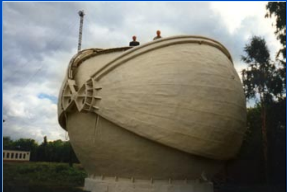
SAZHEN – T OLS shelter
