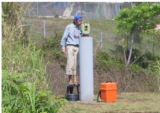
Fig. 8: a total station set on RM-3
