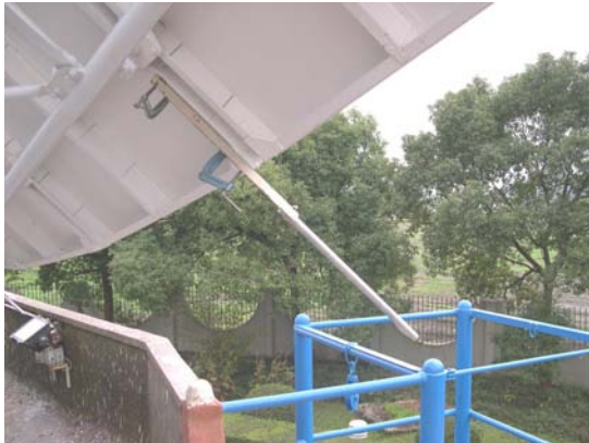
Target placed on the VLBI antenna structure
