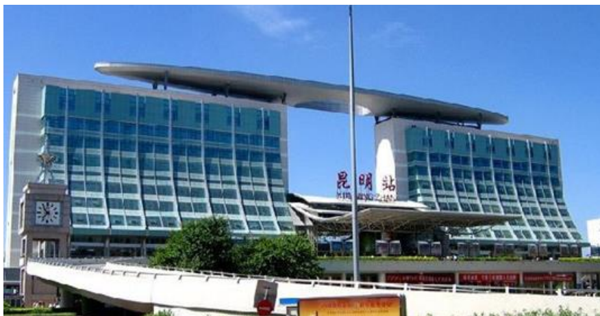
Kunming railway station
