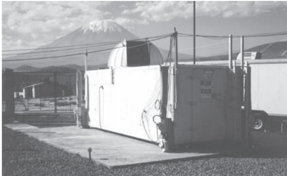
Figure B-1. The TLRS-3 system in Arequipa, Peru.
